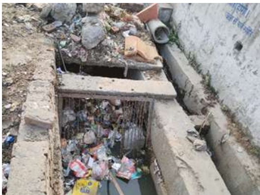
Picture 7-9: Illustration of galvanized Iron Screen at Jagjeetpur I&D Structure
