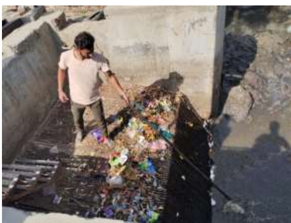
Picture 7-12: Solid waste accumulated at Pandeywala and Kasawaan Nalla I&D Structure
