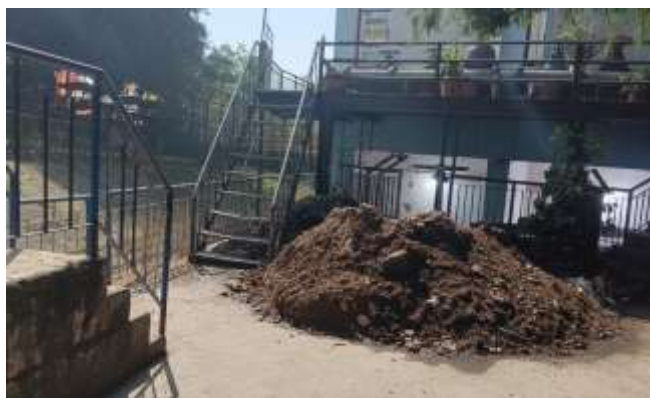
Silt removed from Bhimgoda SPS
