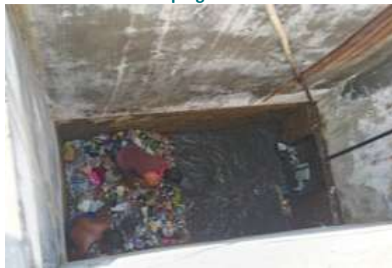
Manual cleaning of Kasawaan SPS
