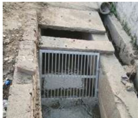
Picture 7-9: Illustration of galvanized Iron Screen at Jagjeetpur I&D Structure
