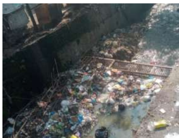
Picture 7-12: Solid waste accumulated at Pandeywala and Kasawaan Nalla I&D Structure
