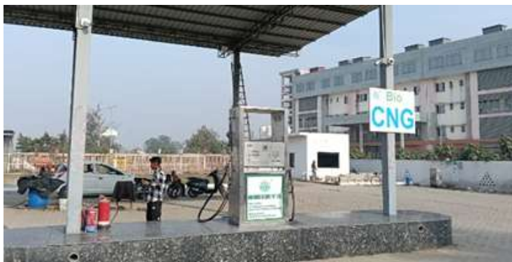
Picture 4-6: Bio-CNG Plant inside Jagjeetpur STP
