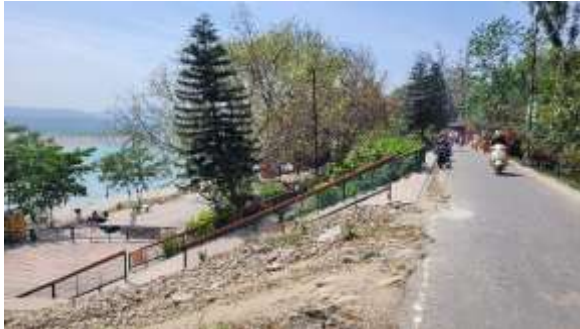
Picture 3-2: Flood embankment along western bank
